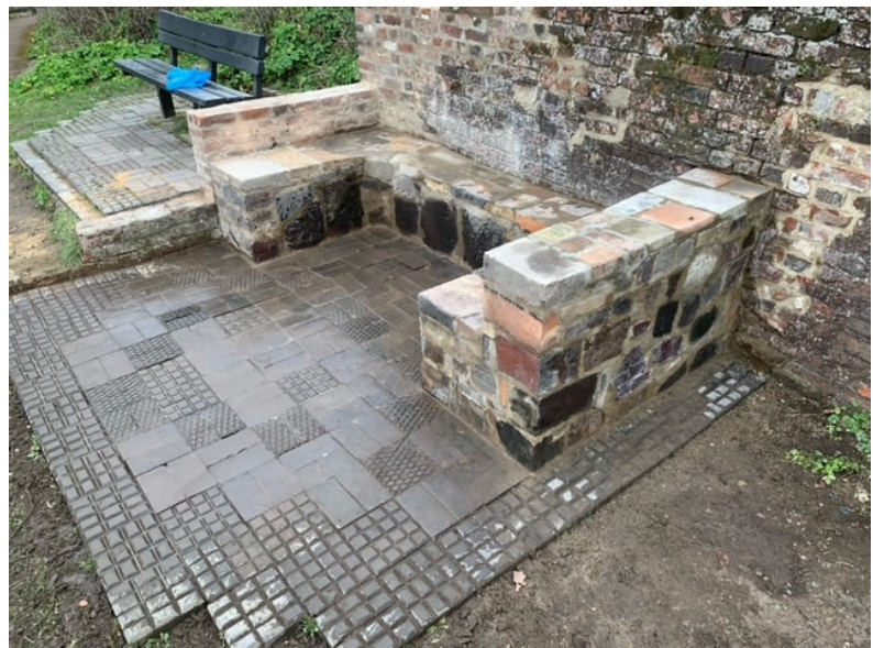
The newly completed seating area on the lower viewpoint. All construction materials were sourced locally from reclaimed bricks and coke oven linings.
